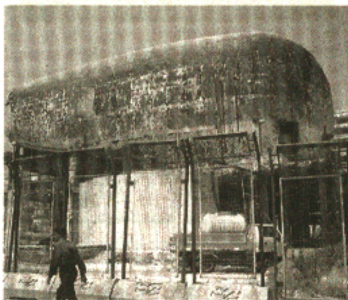
The Beirut City Center Building
